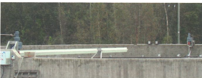
Patented scum gate opens with the help of the scraper flight, releasing the system when the scum scraper is approaching.
