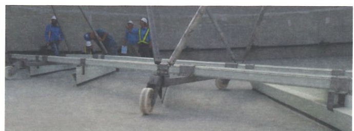
The release system can be adjusted according to the amount of the scum: height of opening gate before scraper approach, length of opening period.
