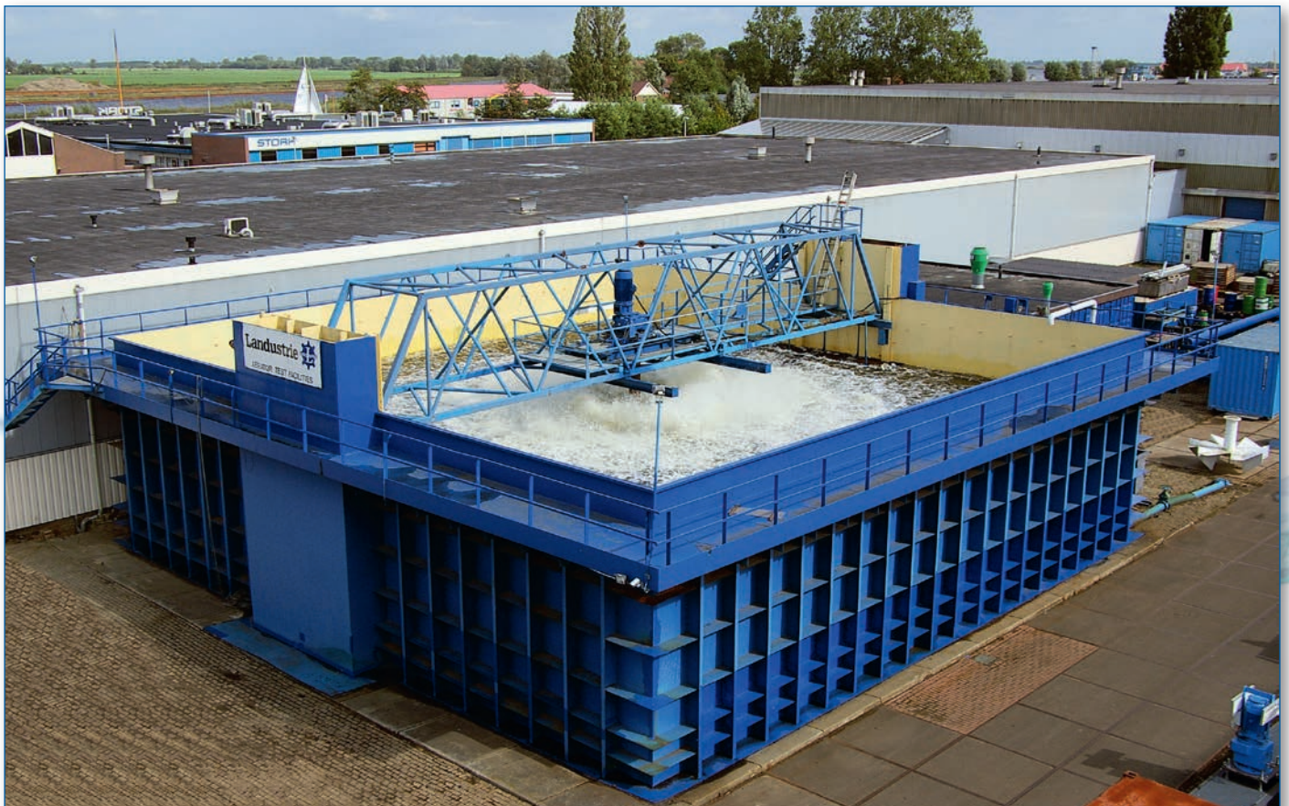
Full scale test basin at Sneek, The Netherlands
