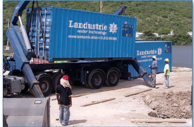
Commissioning at site
