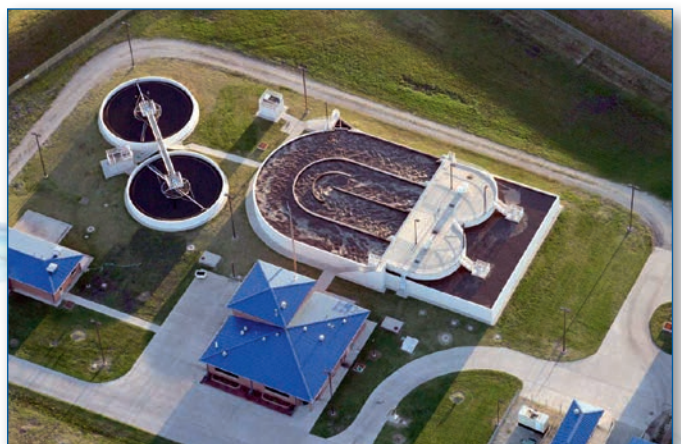
LANDY surface aerator at oxidation ditch
