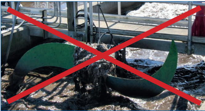
Undesirable clogging of conventional mixers
