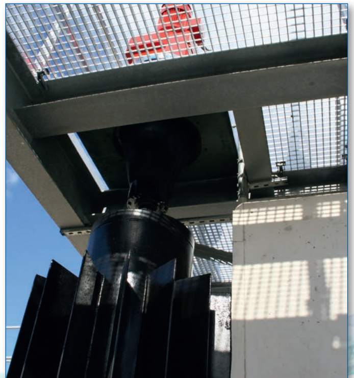
LANDOX flow booster fixed to steel bridge
